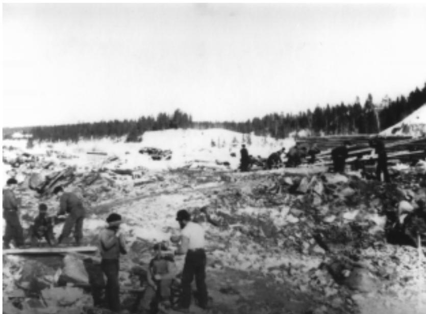
FIGURE 7. Clearing the rapids and building of a twin-faced box boom, probably at the turn of the century (1900), in *Degerforsen* and the eddy just above *Kallholmen*.
